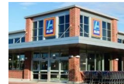
Aldi Buffalo, NY Transcritical CO 2 Booster & Propane
